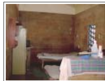
Prisoner cells were being refurbished during the inspection after many years of neglect.
