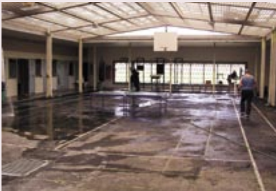
Older parts of the prison though are at a state of considerable decay
