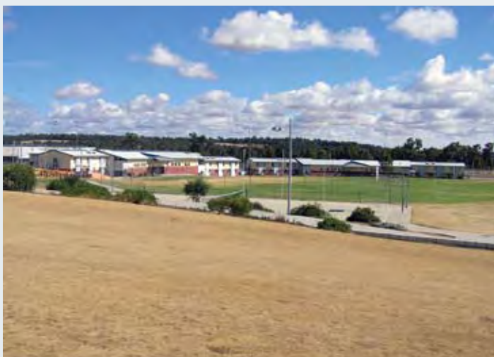
General view of the oval and accommodation units. The view of the hills and trees on the horizon is important for prisoners, particularly the out of country Aboriginal prisoners.
