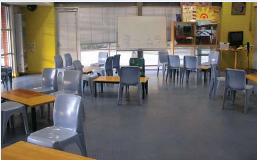
The internal visits room was also need of an upgrade. There were no facilities for outdoor visits and no children’s play area.
