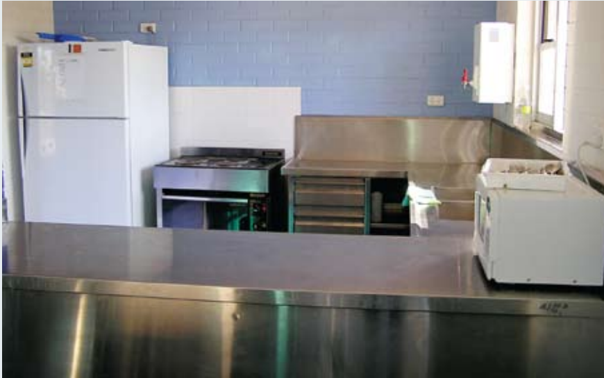
New stainless steel benches and cupboards had been installed in standard accommodation kitchens to replace badly damaged domestic-grade fittings.
