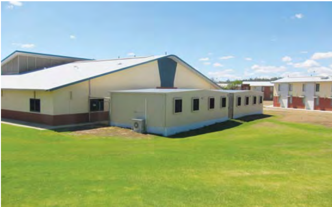
Oscar block: The exterior of Oscar Block showing two transportable units that have been attached to the main building. Further expansion will be needed to accommodate proposed prisoner population increases.
