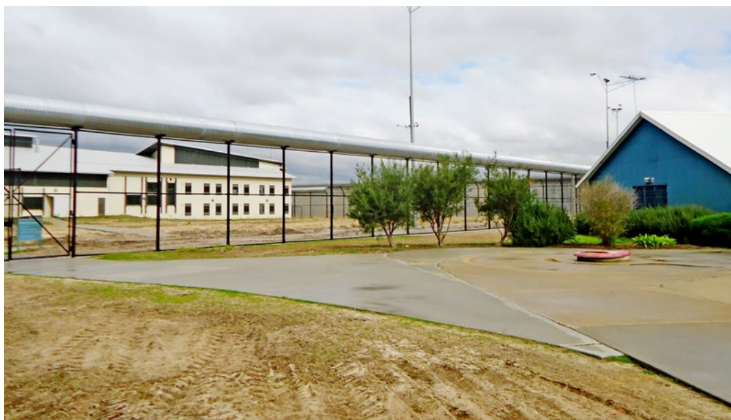
Figure 12: Demarcation fence between Unit 8 at right and the new women's facility.
