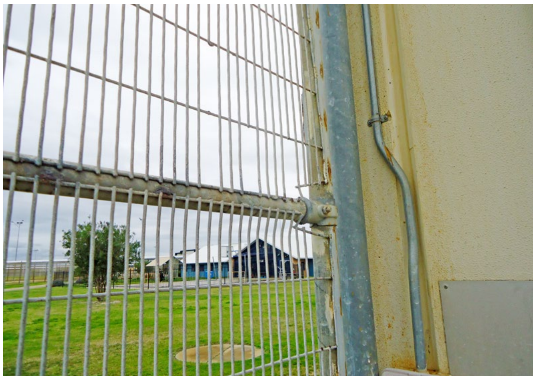
Figure 11: Deterioration in unit fences posed a serious risk.
