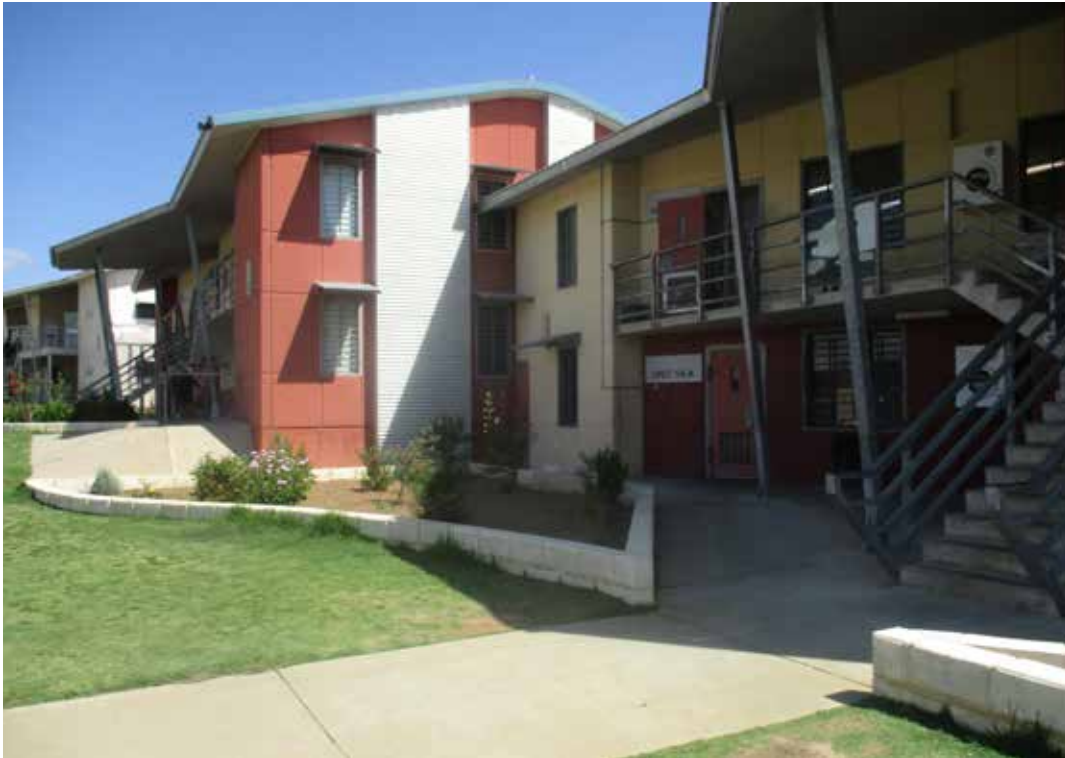
Figure 3: Self-care accommodation units
