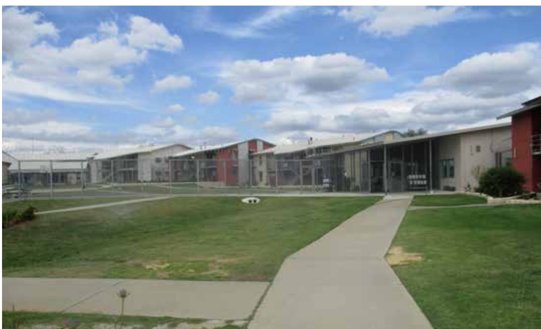
Figure 2: Self-care accommodation units
