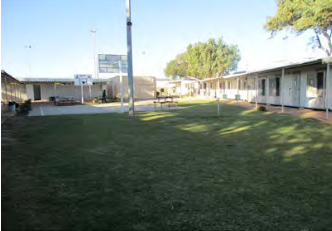
Figure 3: A view across part of Unit Six.
