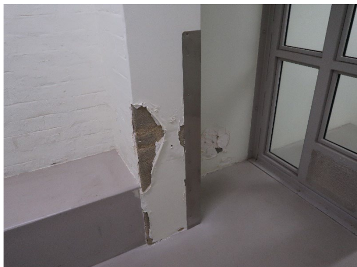
Photo 5: Rising damp evident inside custody cells at the Supreme Court.
