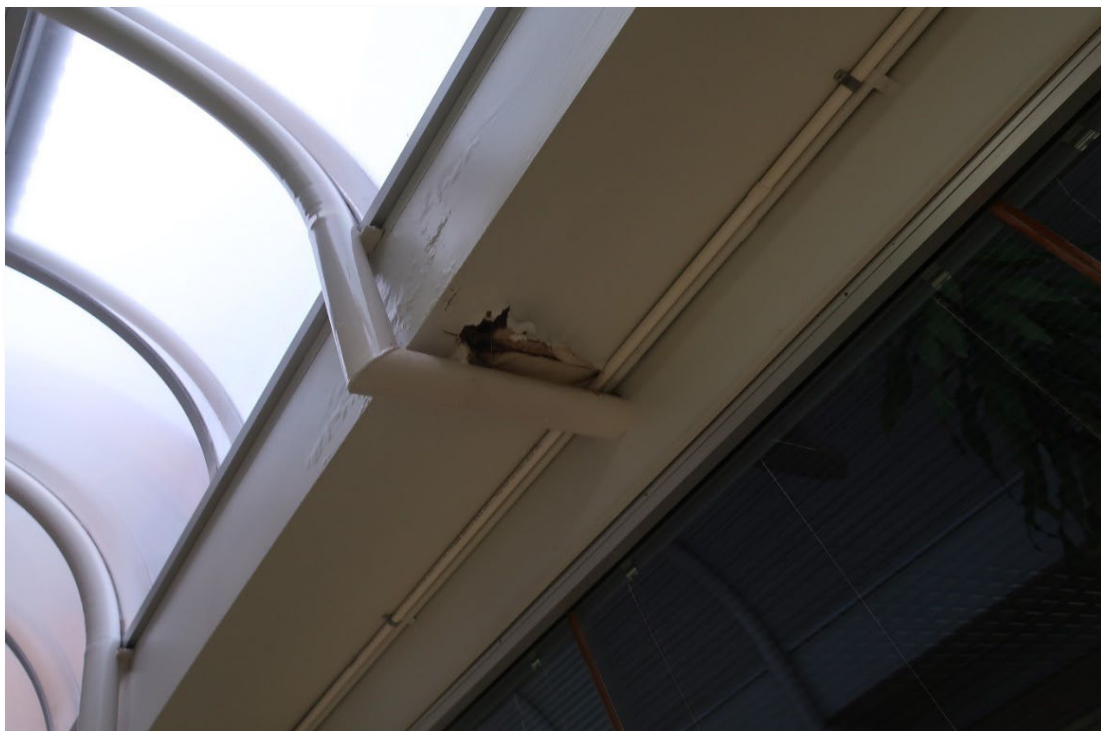
Photo 6: Water leaked from a damaged roof in the administration area.
