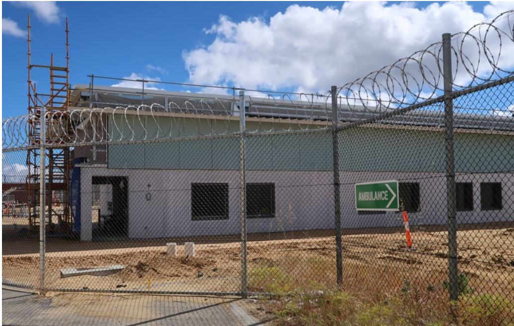
Photo 1: The new Assisted Care Unit was under construction.
