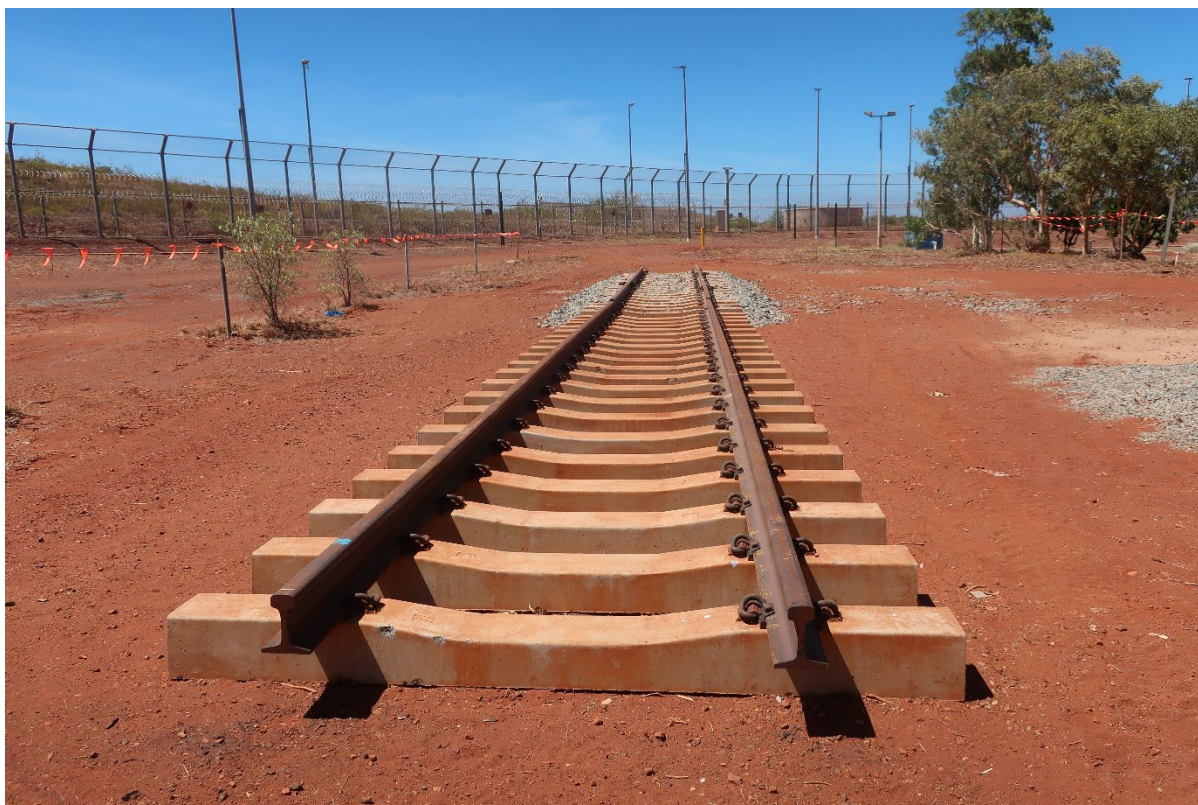
Photo 9: A section of railway track laid in the prison as part of the Bulujari Guma rail infrastructure program.
